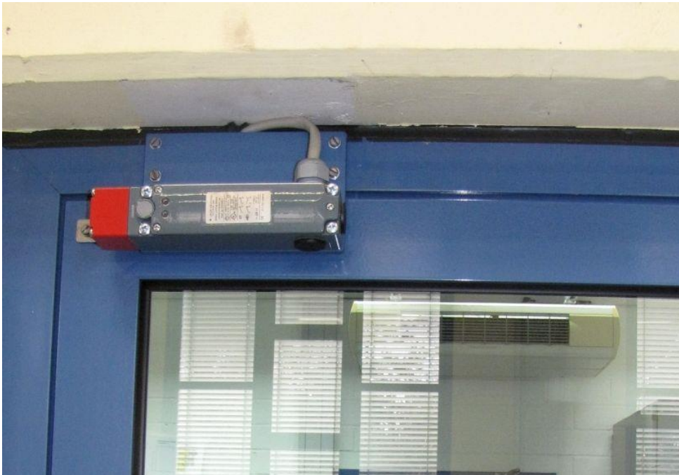
Figure 5. Heavy-duty L200 locking devices were mounted in front of the doors to ensure that no one can enter during the dangerous test.
